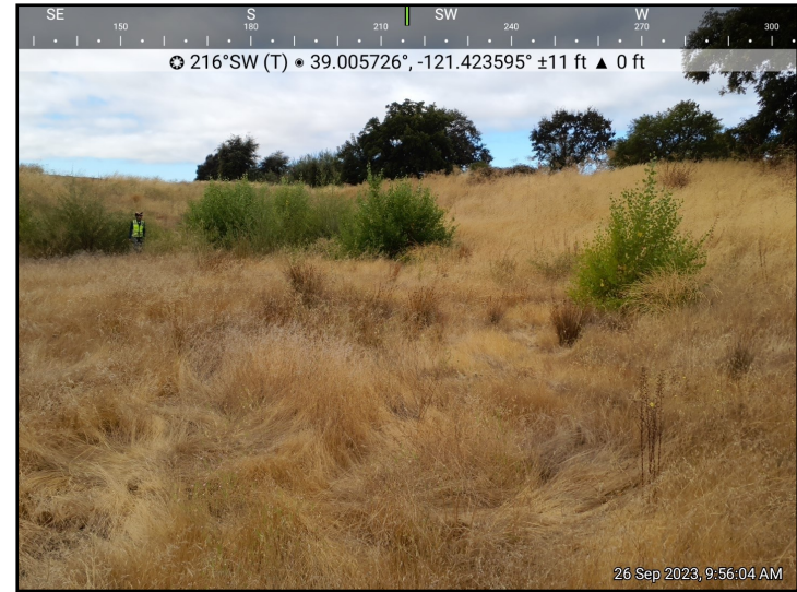
Photo 6: Excavated Detention Pond-Upland
