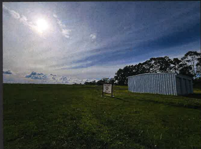
STATION 2 NEW BAY BUILDING
