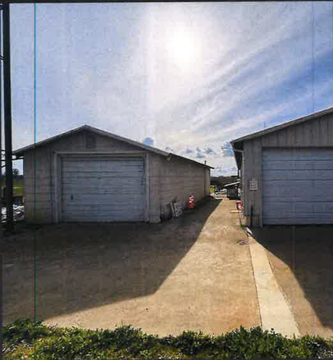
STATION 3 REPAIR/NEW GYM
