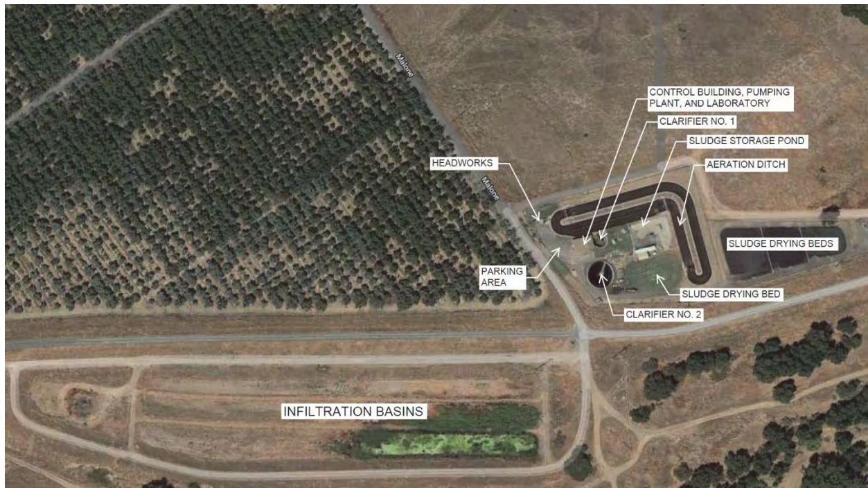
Figure 9-1: Existing City of Wheatland Wastewater Treatment Plant
