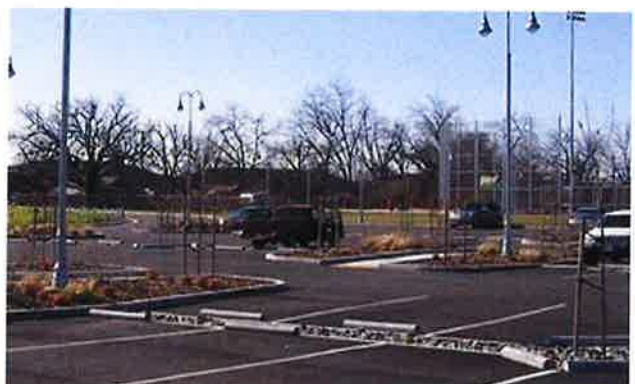
LID - The parking lot's low impact design features waterwise planting and small cobble water collection for first flush and recharge to aquifer.
