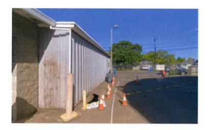
After discovering the hole and void, staff removed a small area of asphalt paving around the original hole which revealed a very large and deep void with tunnels extending beneath the shop building foundation and under the asphalt parking lot into the corporation yard. It appears that surface stormwater has found its way to an abandoned well and has eroded soil through the well.
