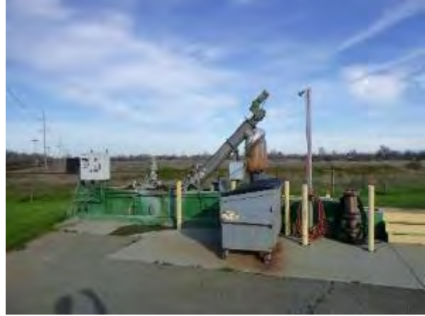
Photo 112 – View to the north, mixing auger and trash collector.
