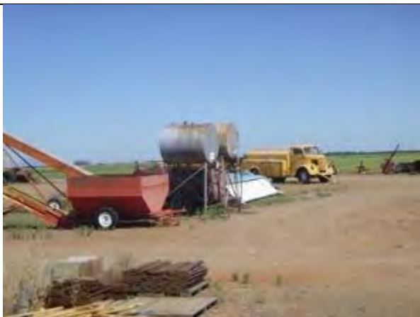
Photo 53 – View to the north of elevated diesel and unleaded gasoline tanks. Minor staining beneath tanks.
