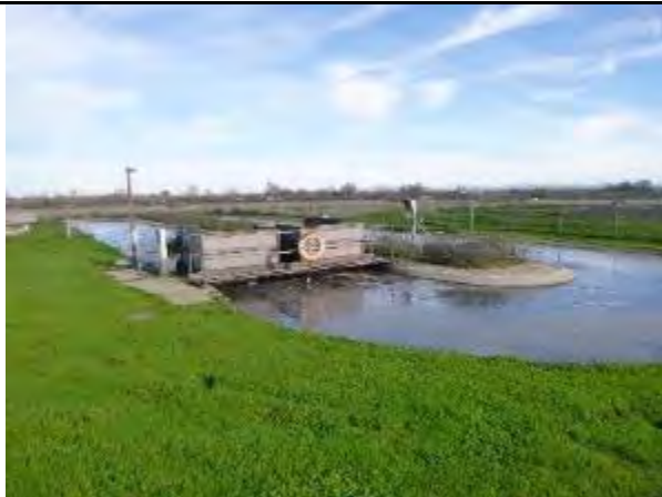
Photo 115 – Aeration Pond with at the Treatment Plant.
