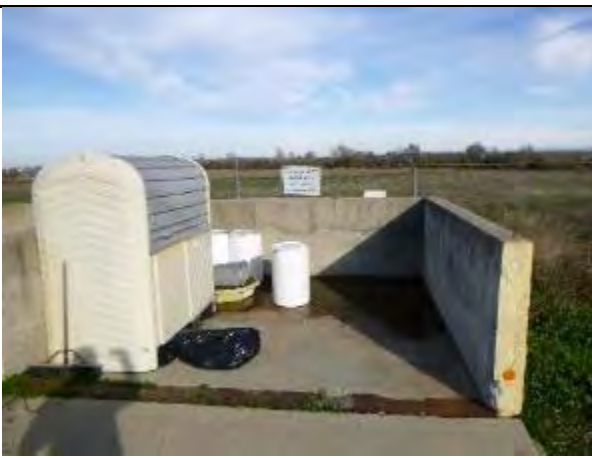
Photo 120 – Hazardous Waste Storage Area with small shed, unused secondary containment and five drums.
