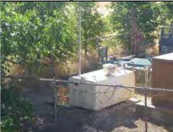
Photo 3 – Emergency diesel fuel tank (250 gallons). No staining or stressed vegetation.
